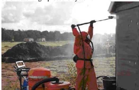
Fig 3. Decontamination of walls by means of a cold-water high-pressure system.
