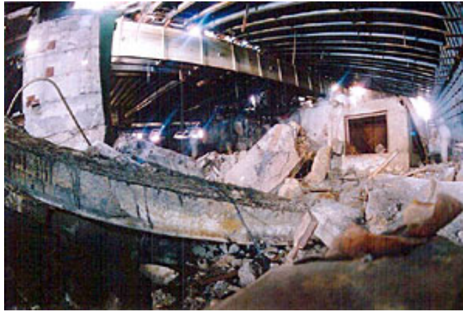
FIG. 6.4. Reactor room of Unit 4 after the accident.
