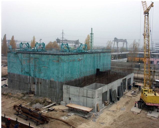
FIG. 6.10. Existing above ground storage facility for solid radioactive waste at the ChNPP Site.
